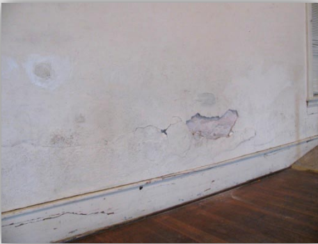
Damaged plaster wall and baseboard
